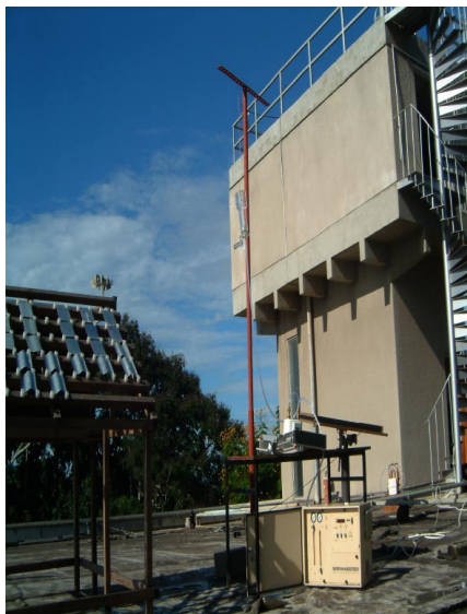
Figure 3. A photo showing a rack of the exposed roof tiles and the PM sampling unit, at site S2.
